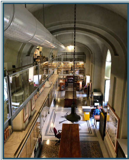
The ventilation system adapted to the rooms of the Prints Cabinet
