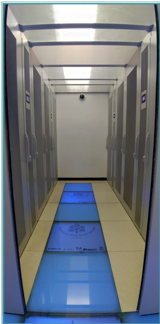
Part of the Data Center of the Library
